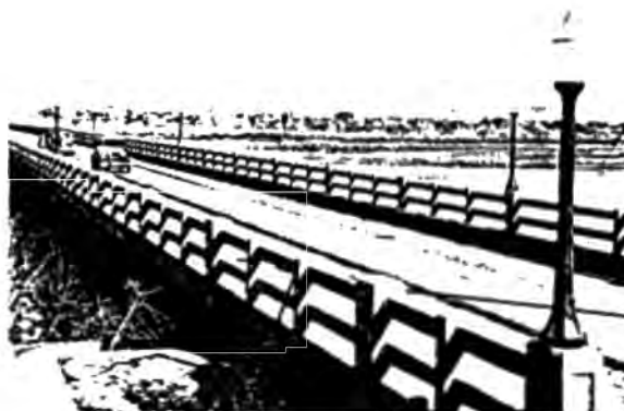
Barelas Bridge Across the Rio Grande at Albuquerque. Completed in 1928, the Barelas Bridge included timber pilings, steel floor beams and a concrete deck. (Highway Department Bridge Files, Inactive)
