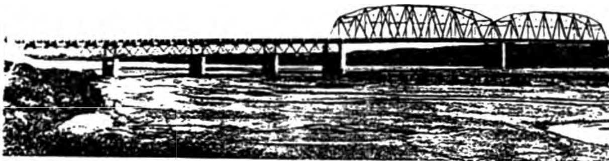
Pecos River Bridge at Fort Sumner. Completed in 1927, the Pecos River Bridge included two through truss spans of 252 feet each and four deck truss spans of 75 feet each. ( N.M. Highway Journal , September 1927, p. 8)
